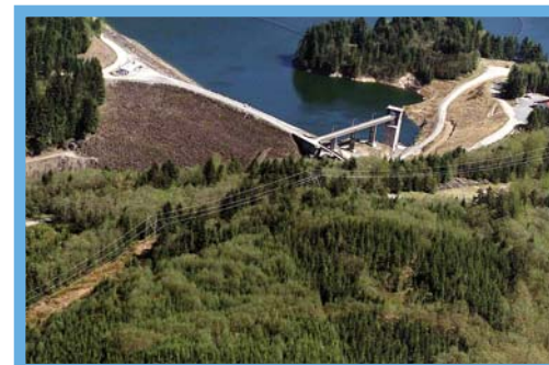
Howard Hanson Dam in Tacoma's Green River Watershed
