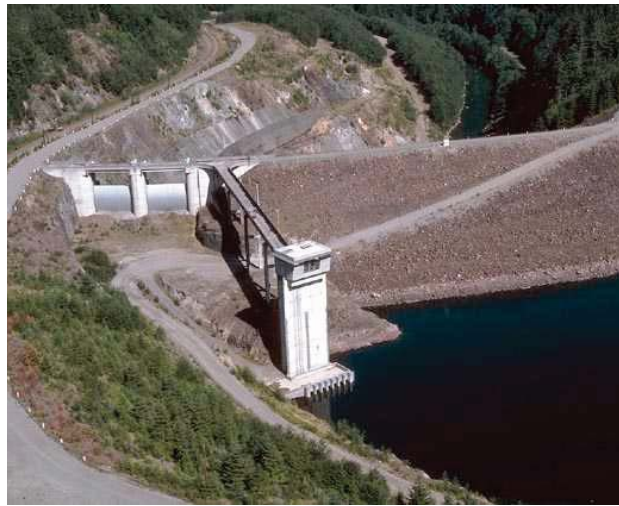
The Howard A. Hanson Dam originally named the Eagle Gorge Dam is located on the Green River, 21 miles east of Auburn, Washington.
